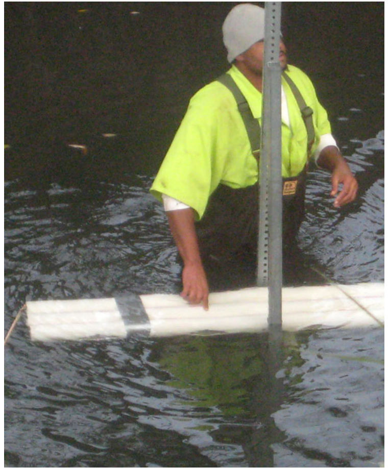
5a) PLACE PIPE(S) IN SUPPORT STRUCTURE . . .
