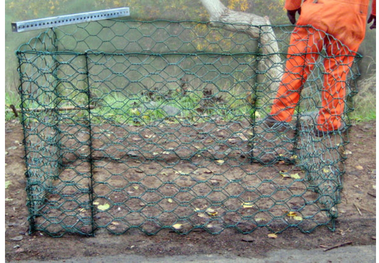
3) CAGE CREATED FOR INTAKE END OF PIPE(S)
