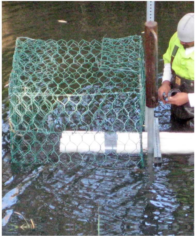
8) SECURE CAGE AT INTAKE END OF PIPE(S)
